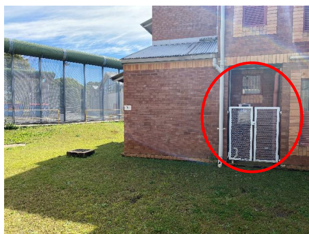
A gas hot water system attached to the wall of one of the cells in the southwest corner of the site
